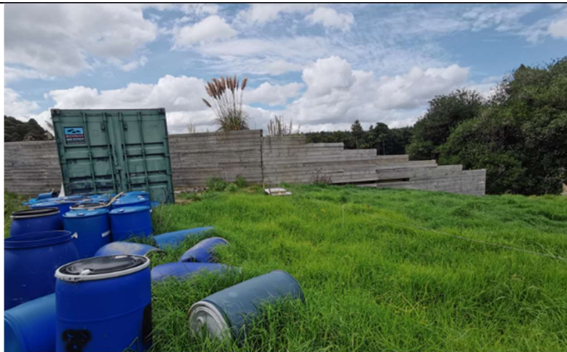
Figure 4.5: Existing retaining wall of 2m height
