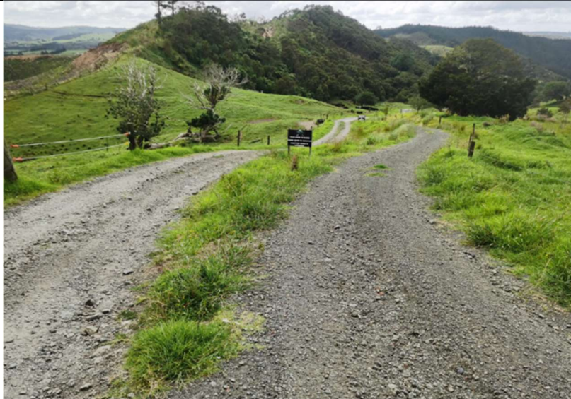
Figure 4.4: Metal access driveway from Tuhirangi Road
