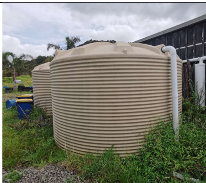
Figure 4.6: Existing 25,000L rainwater tanks
