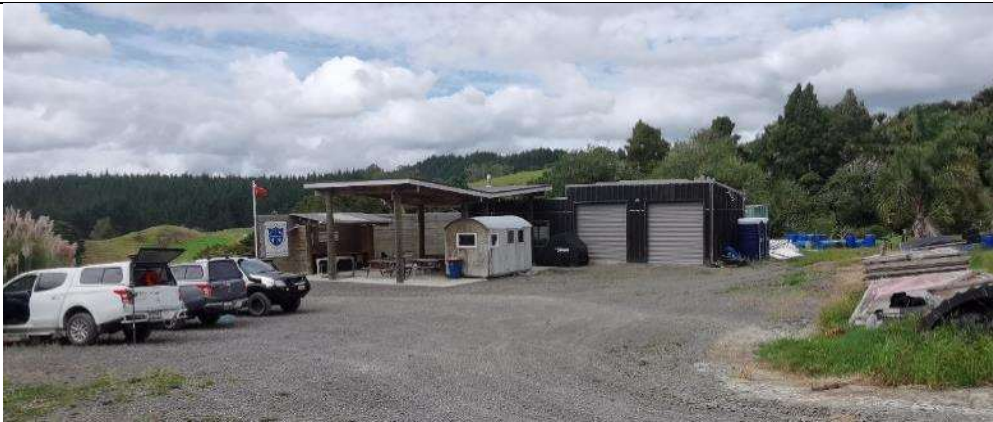
Figure 4.8: Existing ancillary structures including administrative box, waiting area and port-a-loos
